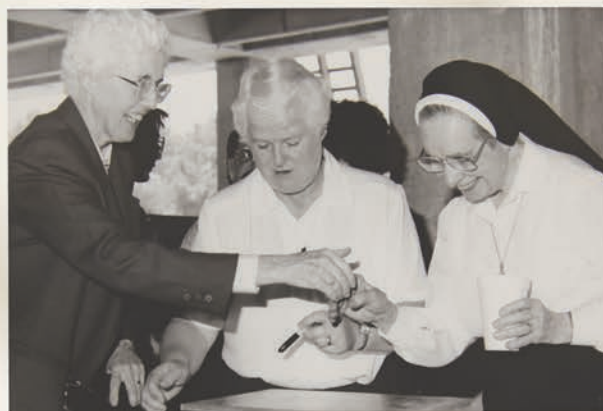
June 1993 Topping Out Ceremony for new St. Michael Health Care Center
